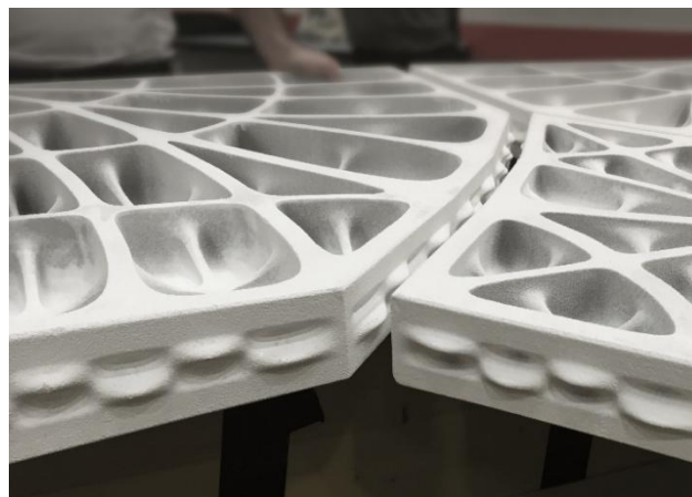
Fig. 3–Dry joint between blocks.
